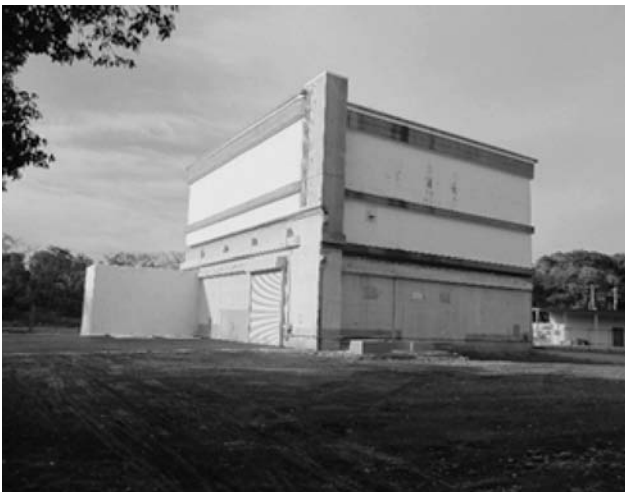
Fig. 30 HTR from north east side after demolishing
