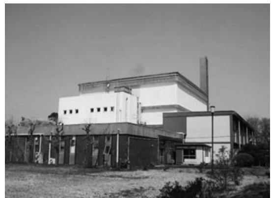
Fig. 27 HTR from south side before demolishing
