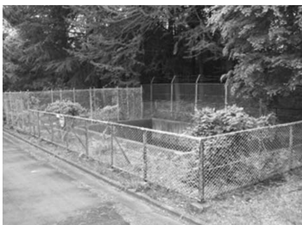
Fig. 18 Dilution pond before demolishing
