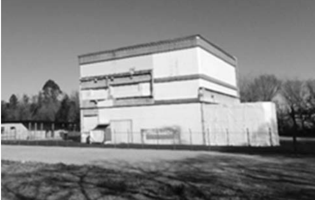
Fig. 28 HTR from south side after demolishing
