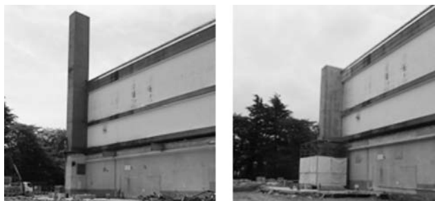
Fig. 17 Stack before and after dismantling
