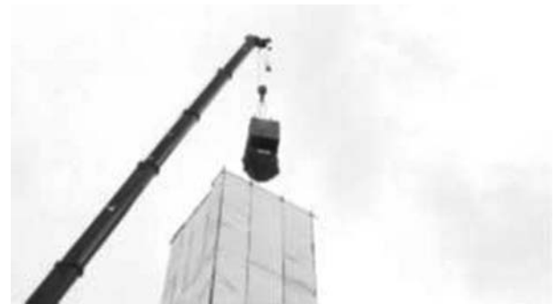
Fig. 15 Dismantling process of stack
