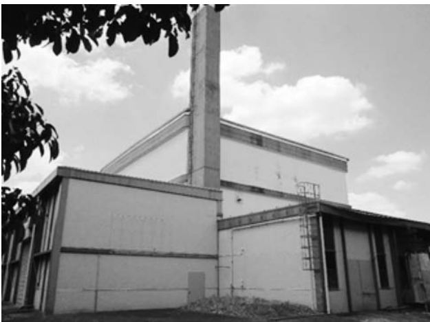
Fig. 29 HTR from north east side before demolishing
