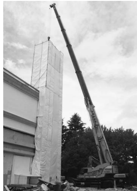
Fig. 14 Cutting process of stack
