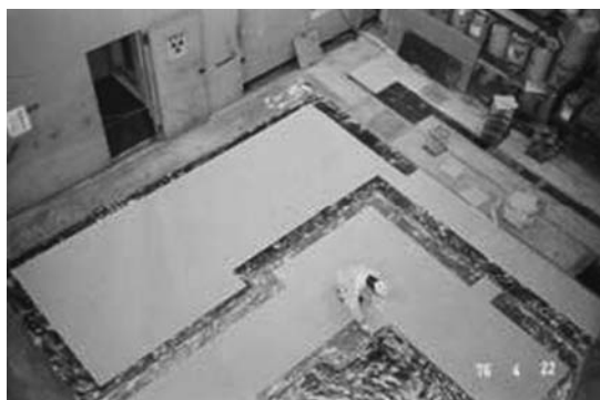
Fig. 11 Changing tiles in the reactor building
