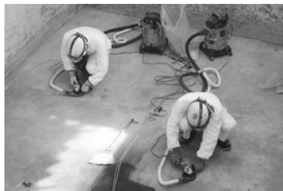
Fig. 20 Removing inside of dilution pond
